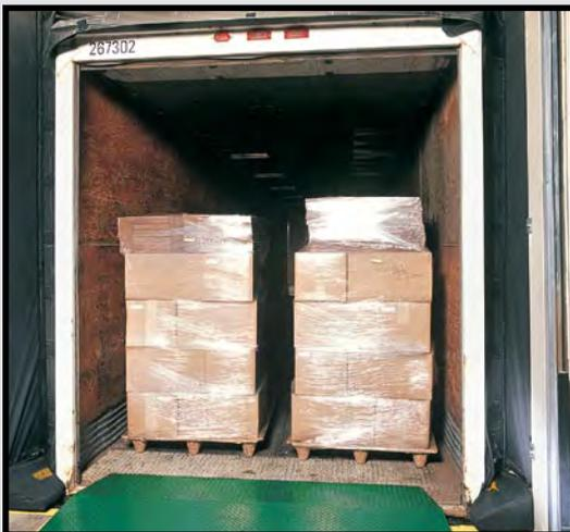
When the trailer is backed into position, no foam or fabric impedes the doorway, providing clear and unobstructed access to the trailer.
