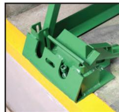
The installer adjusts the leveling bolts on the front and rear supports using a standard 1/2" square head socket.
